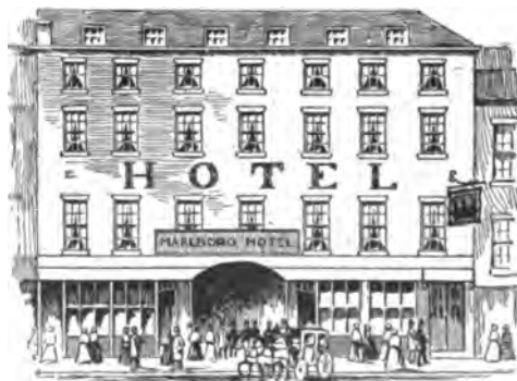
MARLBORO HOTEL. SHOWING PASSAGEWAY TO THE MARLBORO CHAPEL.
